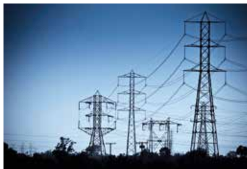
Pylons and high voltage lines providing transmission of electricity
