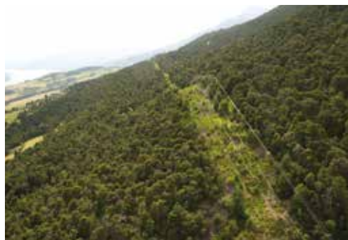
Safety corridor along high voltage lines
