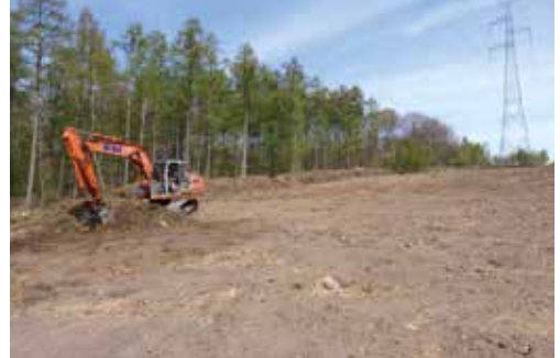
2. Restoration of a dry moor by tillage
