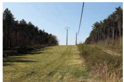
"Mixed" corridor with high and low voltage lines
