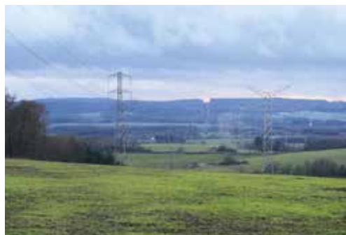
High voltage lines in an agricultural environment
