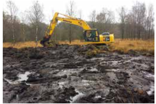
Restoration of a peat bog by tillage and windrowing
