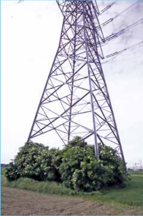
Foot of pylon developed in farm field
